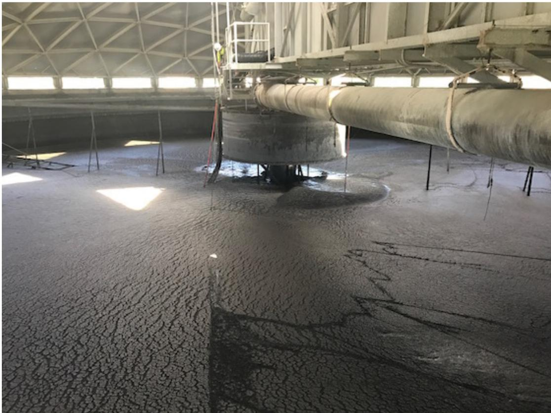
U.S. Submergent Technologies is currently performing sand and grit removal at a wastewater treatment plant in Orlando, FL, which requires confined space entry.
